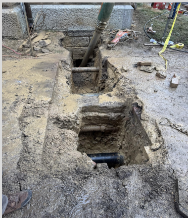
Excavation For Water Tap 1/31/25
