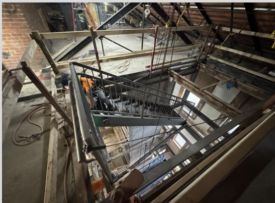
Egress Stair Installation 1/31/25
