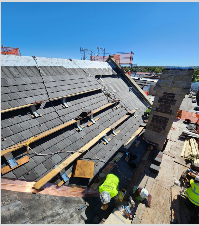
West Elevation Roofing 10/11/24
