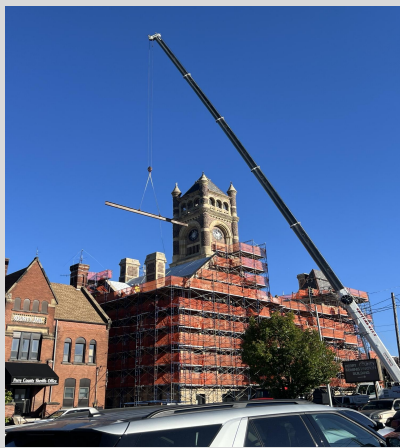
Scaffolding Beam Removal 10/7/24
