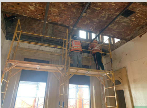
Steel Decking Install 10/11/24
