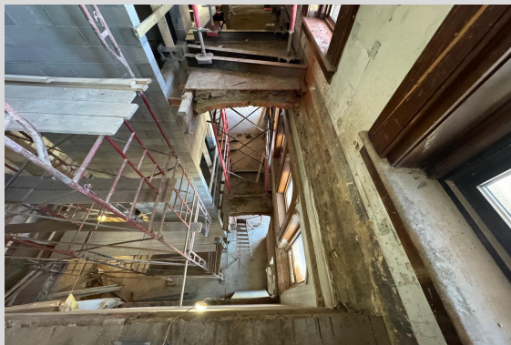
Jack Arch Demo For New Egress Stair 10/18/24
