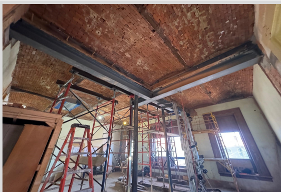
Magistrate Hearing Room Steel Install 10/18/24
