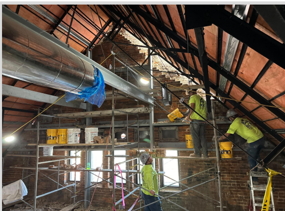
North Gable Brick Wall Repair 10/4/24
