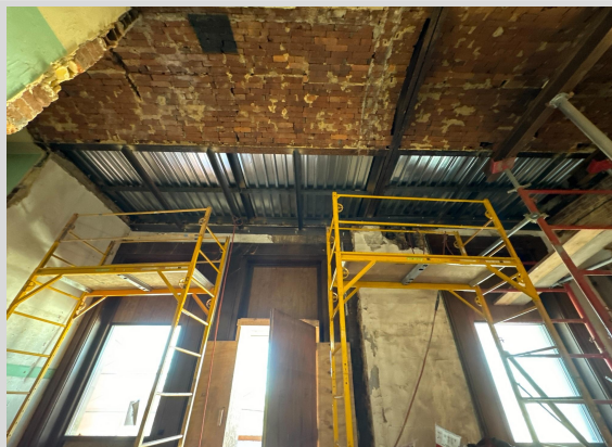
2nd Floor Steel Decking 10/4/24
