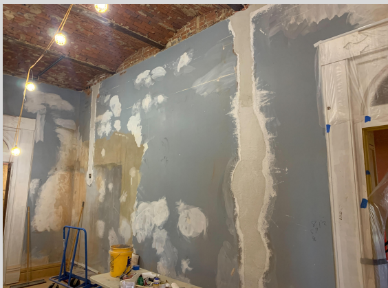
Probate Courtroom Plaster Repair 10/4/24
