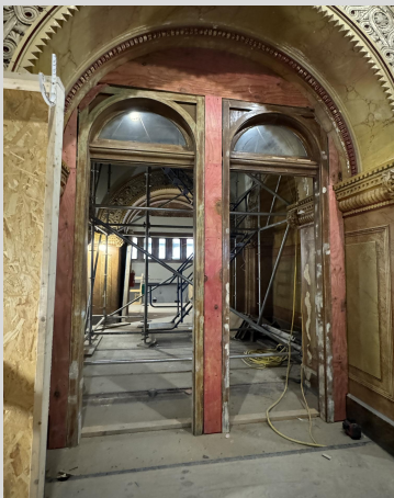
2 nd Floor Opening Build- Out 11/22/24
