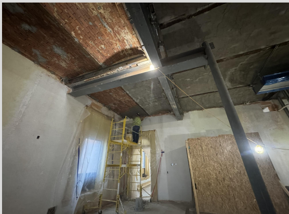
Brick Arch Parge Coating 11/22/24
