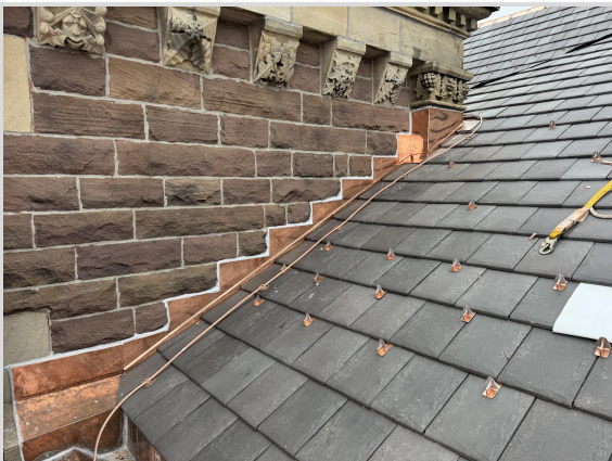
Copper Roof Flashing Install 11/27/24
