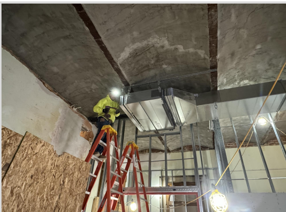
1st Floor HVAC Duct Install 11/27/24
