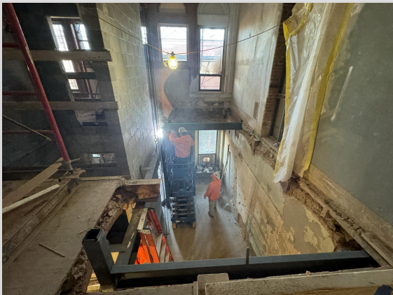
Egress Stair Steel Install 11/8/24
