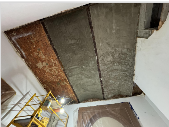
1st Floor Brick Arch Parge Coating 11/8/24
