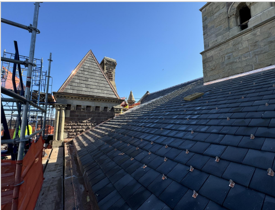
North Elevation Roofing 11/8/24
