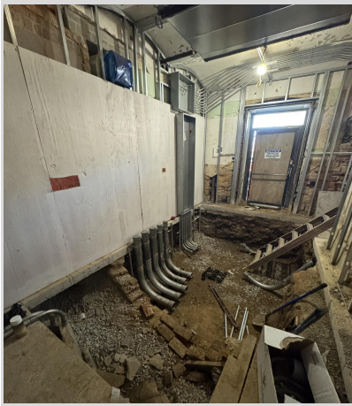
Permanent Power Excavations 12/13/24
