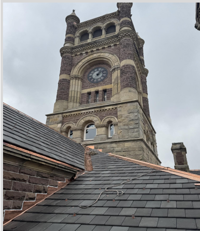
New Clock Tower Window Install 12/20/24
