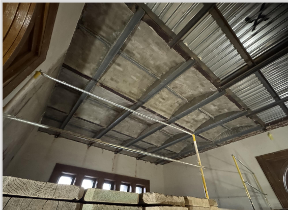
2 nd Floor Arch Stabilization 12/20/24
