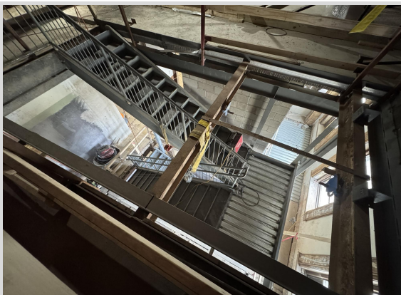
Egress Stair Installation 2/7/25
