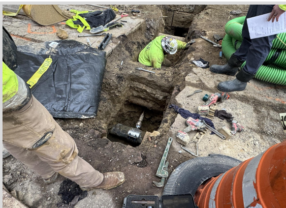
Water Main Tap 2/7/25
