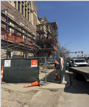
South Elevation Scaffolding Teardown 3/14/25
