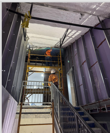
Egress Stair Framing 3/14/25
