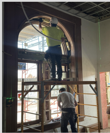
1 st Floor Window Install 3/14/25
