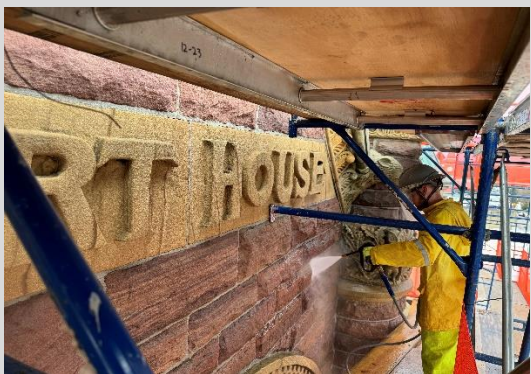
East Elevation Stone Cleaning 3/14/24
