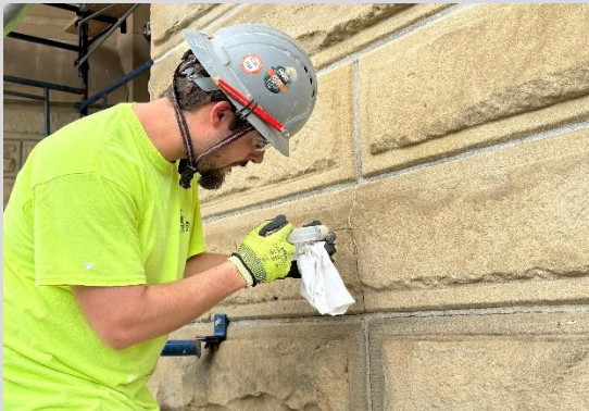
South Elevation Stone Grout Patching 3/14/24
