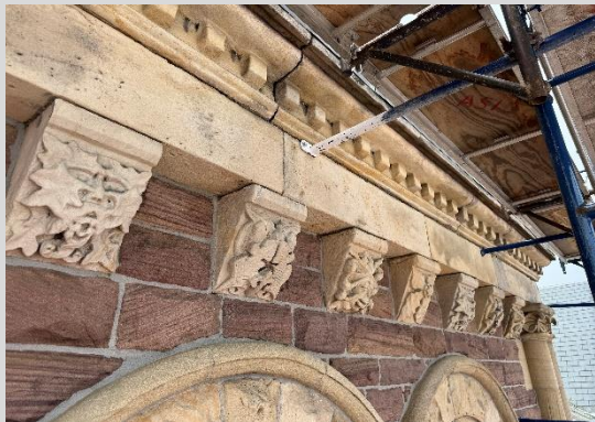
North Elevation Mortar Removal 3/14/24
