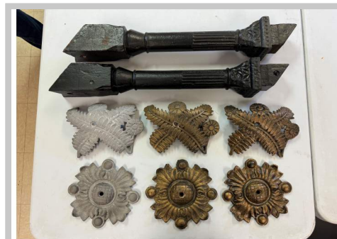
Historic Stair Samples 3/22/24 Top: Original Painted Baluster Left To Right: Sandblasted Originals, Painted Originals, & Painted New Openings
