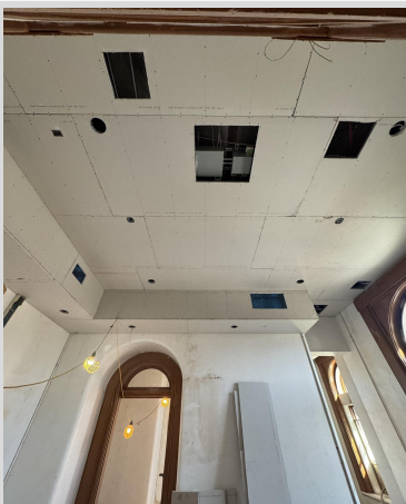
1 st Floor Ceiling Install 4/19/25
