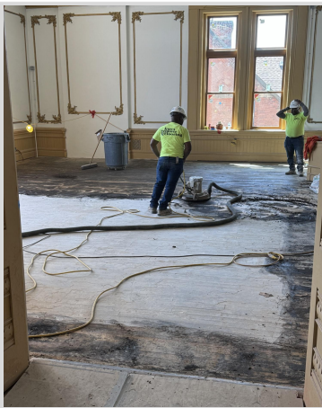
2 nd Floor Courtroom Prep 4/19/25
