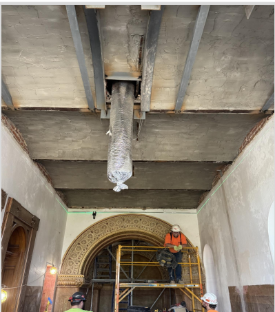
2 st Floor Ceiling Framing 4/25/25
