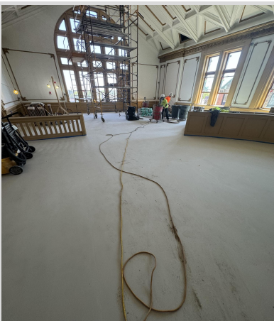
2 nd Floor Courtroom Floor Fill 4/25/25
