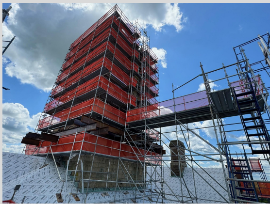
Bell Tower Scaffolding 5/10/24
