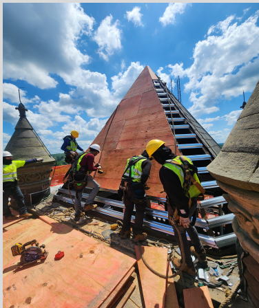
Clock Tower Roof Sheathing 5/17/24
