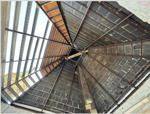
Exposed Clocktower Roof 5/31/24
