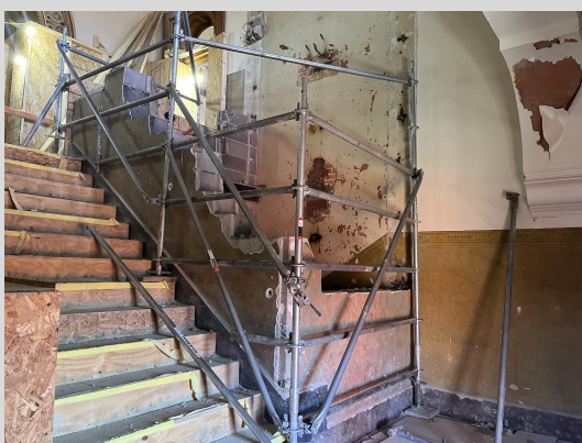
Elevator Shaft Demo 5/31/24
