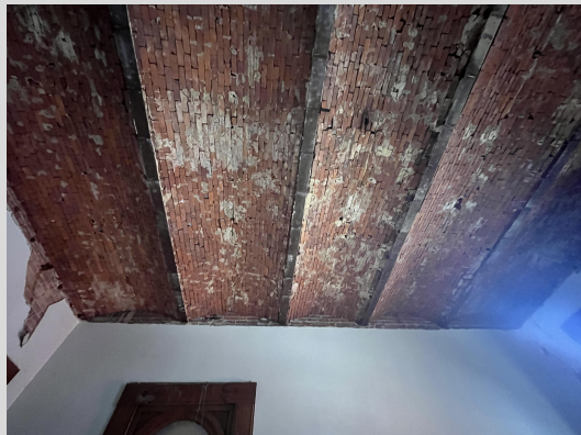
First Floor Plaster Ceiling Demo 5/30/24
