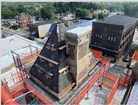
Finished Tile Installation 6/20/24
