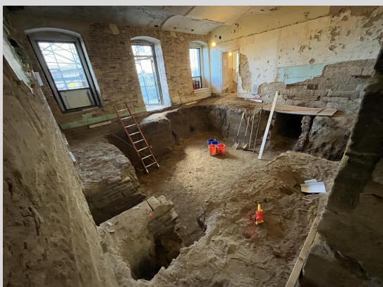
Elevator Footer Excavation 6/21/24
