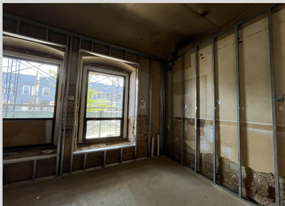
Ground Floor Metal Stud Framing 7/26/24
