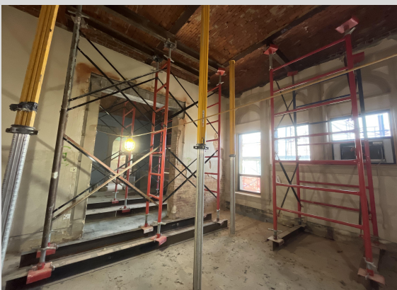
First Floor Shoring 7/26/24
