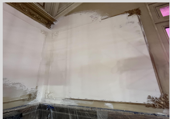
Second Floor Courtroom Plaster 8/1/24
