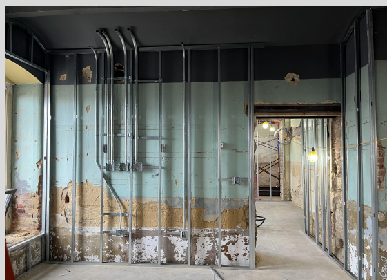
Ground Floor Framing 8/1/24
