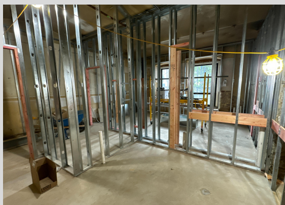
Ground Floor Wall Blocking 8/16/24
