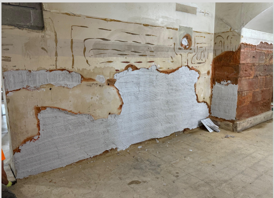
Ground Floor Plaster Repair 8/16/24
