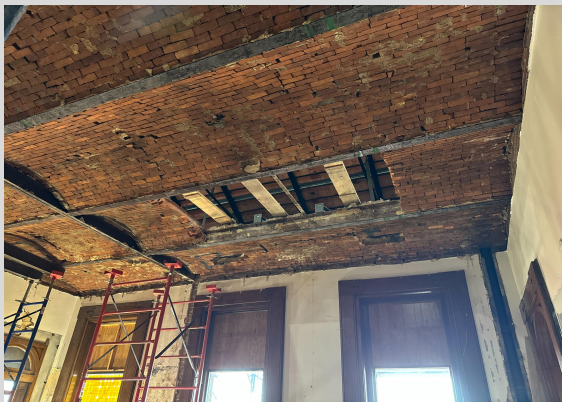
Egress Stair Floor Demo 8/16/24
