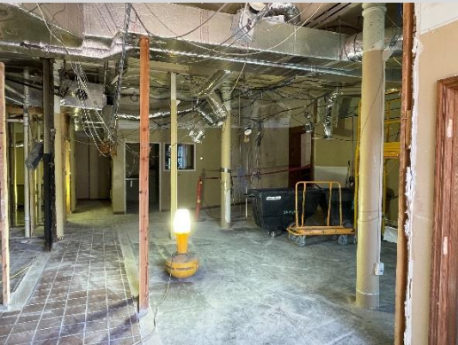
Demolition Ongoing Ground Floor
