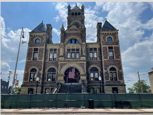
Temporary Fence Installed
