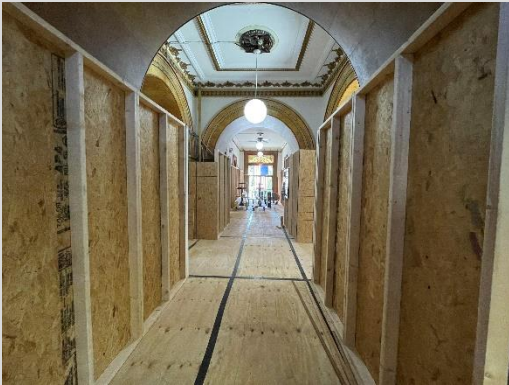
Wall Protection Installed 1 st Floor
