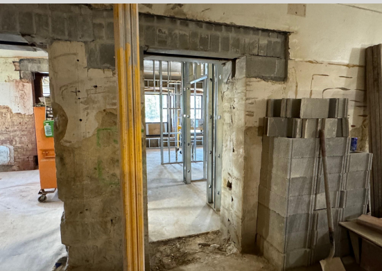
Ground Floor Opening Demo 8/9/24
