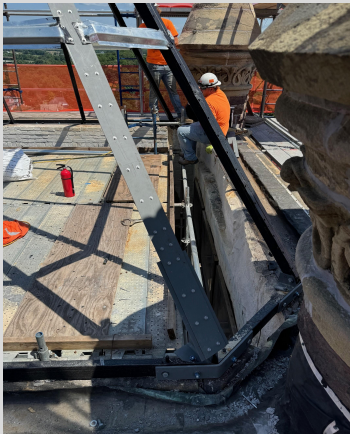
Clock Tower Steel Install 8/8/24
