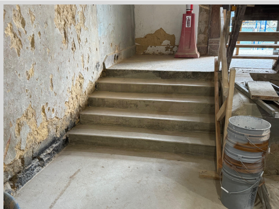
Concrete Stair Install 9/20/24
