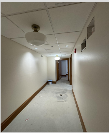
Ground Floor Lighting Install 7/11/25
