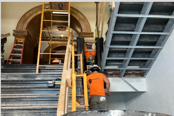
Historic Stairwell Newel Post Install 7/25/25
