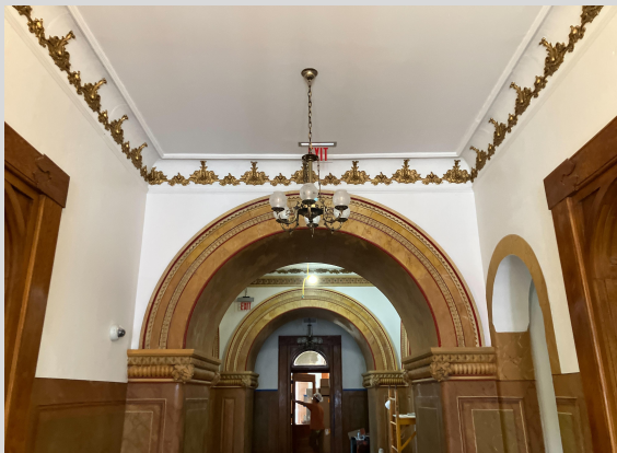
1st Floor Chandelier Install 7/25/25
