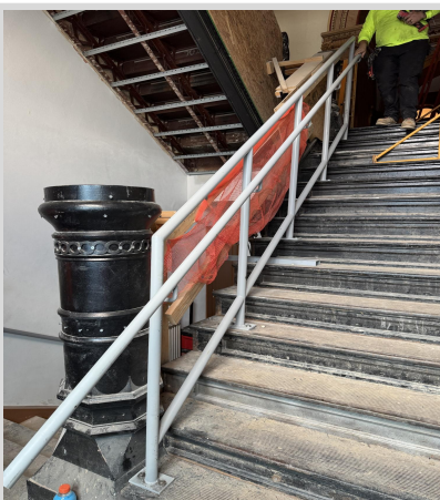
Historic Stairwell Handrail 7/25/25
