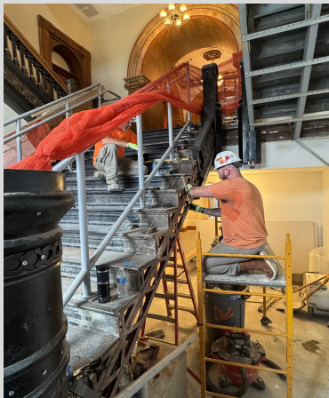
Historic Stair Handrail Install 8/8/25
